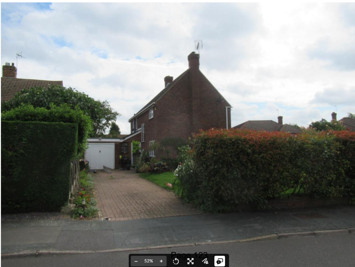
Side elevation and garage of No. 1 Sefton Close with No. 16 adjacent to the left of picture
